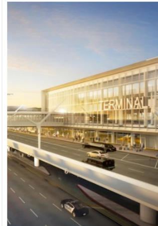
LAX Terminal Cores and APM Interface Project, Los Angeles, CA
