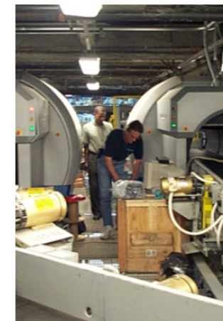
LAX Gate Renovation & Baggage Screening, Los Angeles, CA
